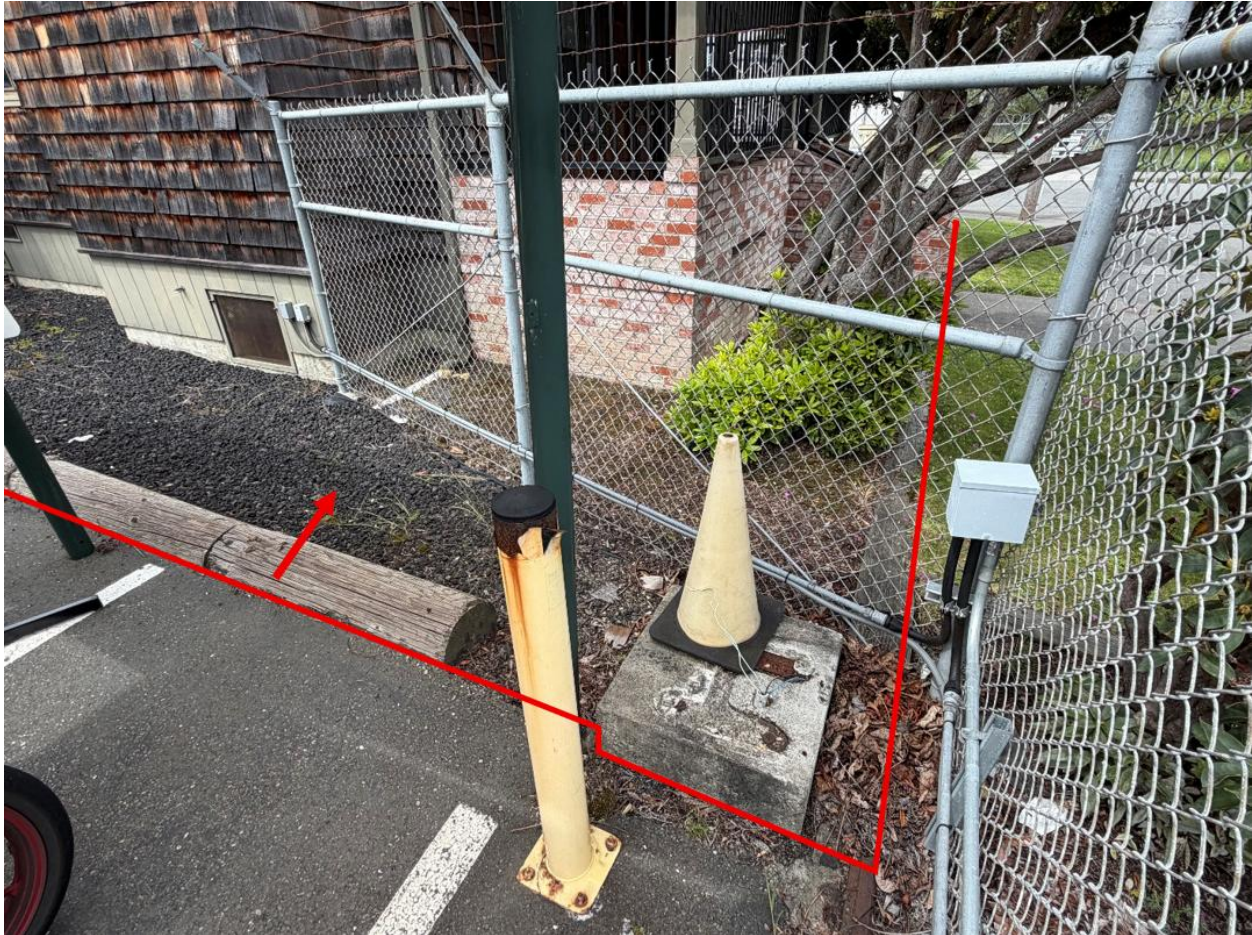
Figure 1: Southeast Edge of Demolition
