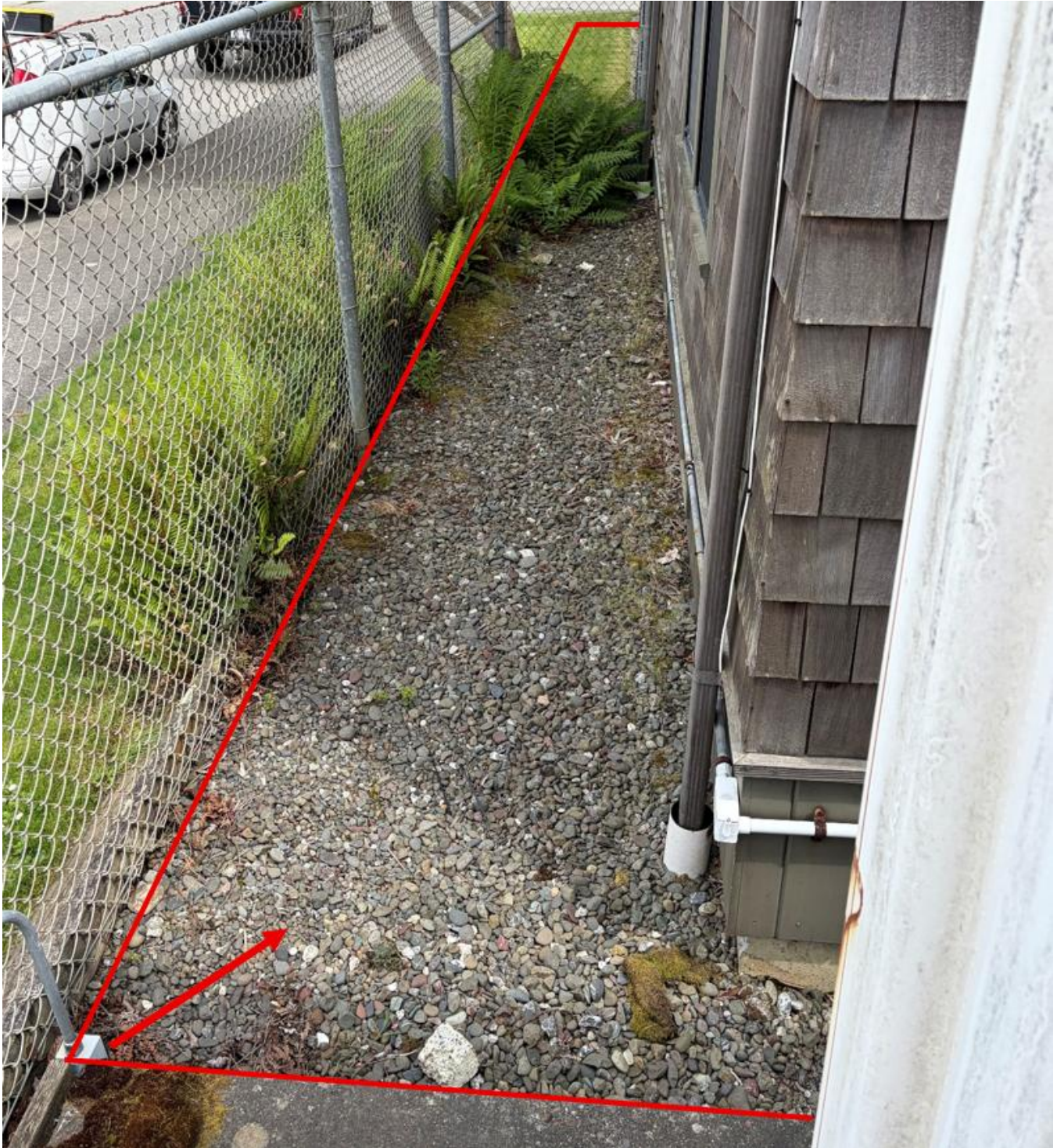
Figure 4: Northwest edge of demolition facing East
