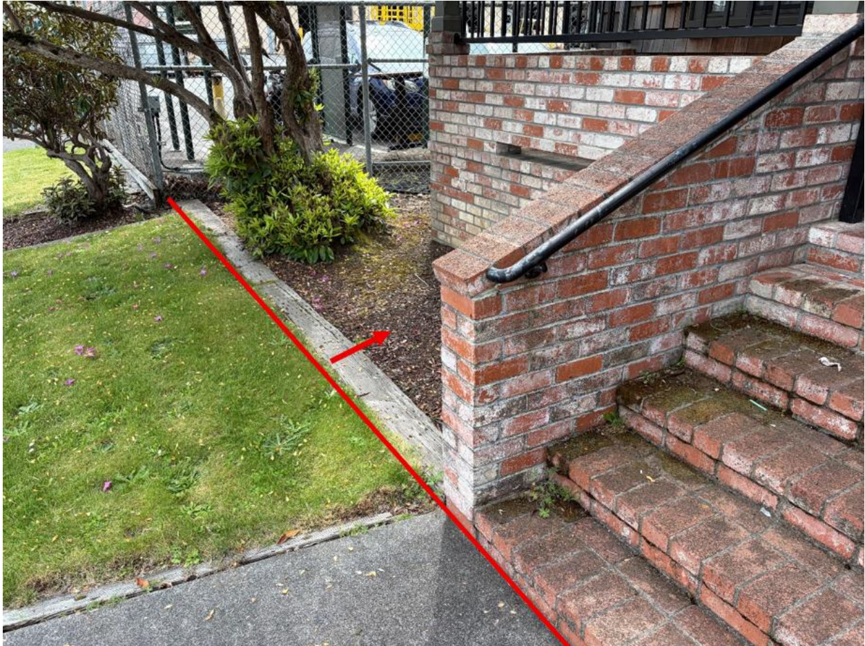
Figure 2: East edge of demolition facing south
