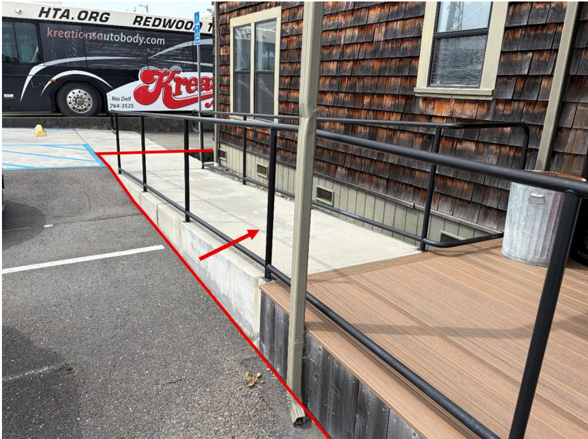
Figure 6: South Edge of Demolition Facing West
