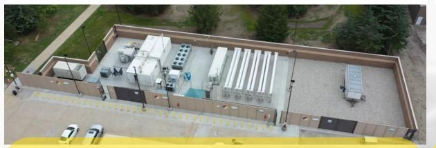
STATION SIZE – 1 MW electrolysis system PRODUCTION – 420 kg per day via Electrolysis TARGET PERFORMANCE – 15 min fills FOOTPRINT – 6,000 sqft. ACTIVELY OPERATING & MAINTAINING
