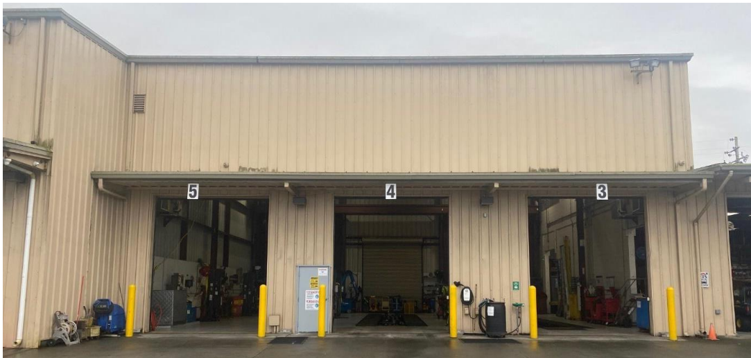
Figure 8: Maintenance bays to be retrofitted at HTA’s corporation yard.
